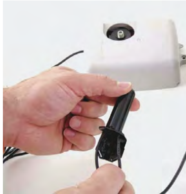
Figure 10 – Splice Tube
