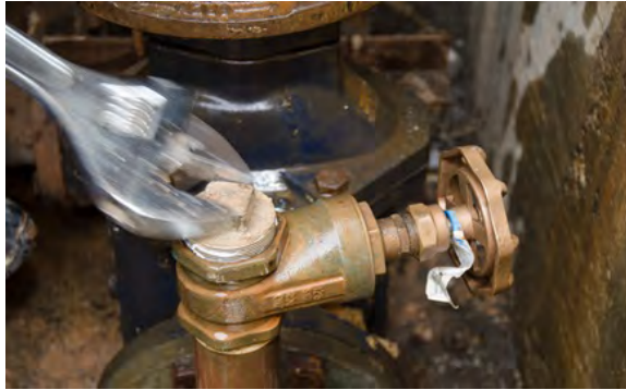
Figure 4 – Remove Test Plug
