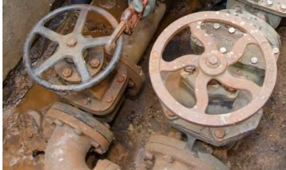
Figure 16 – Bypass Valve
