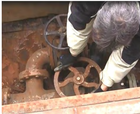
Figure 9 – Inlet Valve
