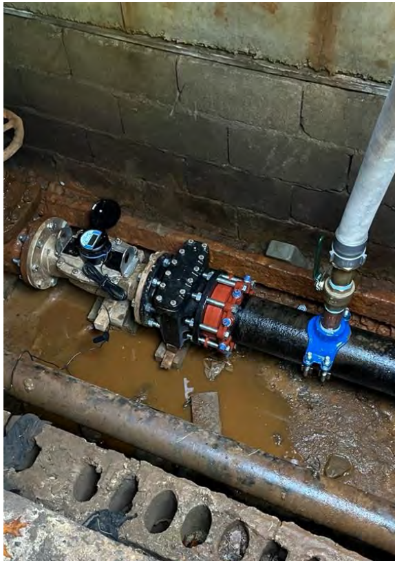
Figure 5 – Connect the Fire Hose to Meter Under Test
