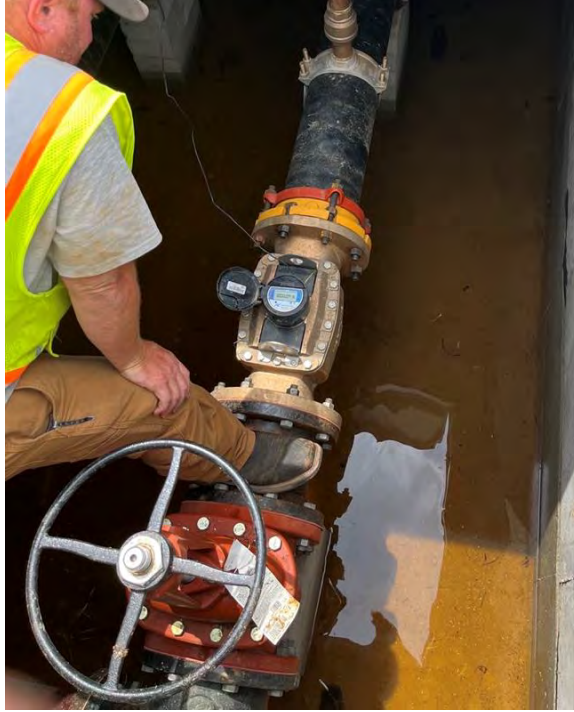
Figure 7 – Take the Initial Read from the MACH 10 ® Display
