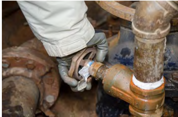
Figure 13 – Test Riser Valve Attached to Meter Under Test
