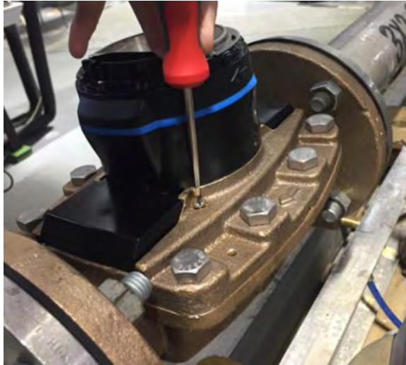
Figure 21 – Turn the Bleed Screw
