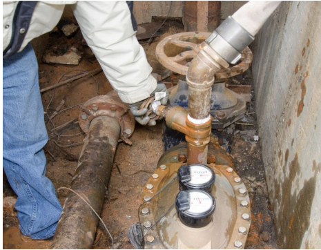
Figure 11 Opening the Test Riser Valve
