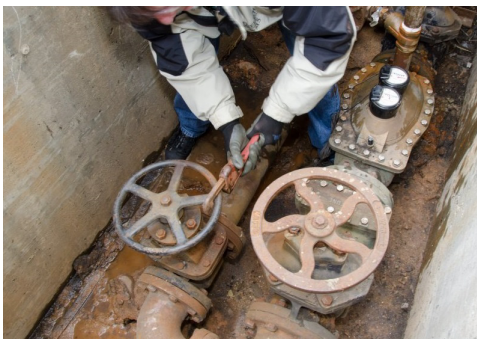
Figure 9 Opening the Bypass Valve
