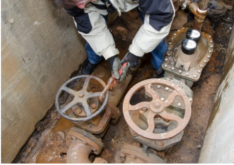
Figure 31 Bypass Valve
