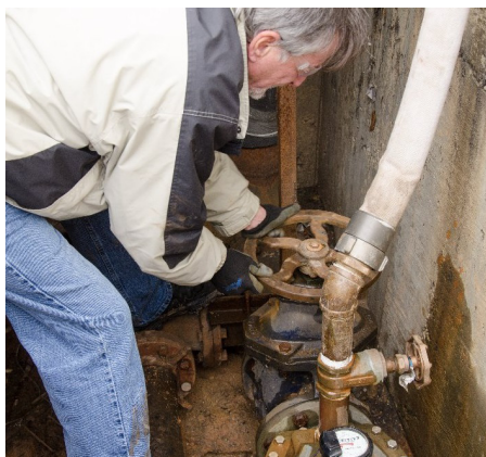
Figure 13 Shutting the Outlet Valve
