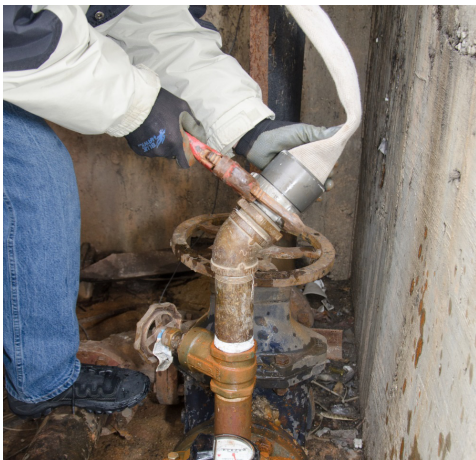
Figure 7 Tighten the Connection
